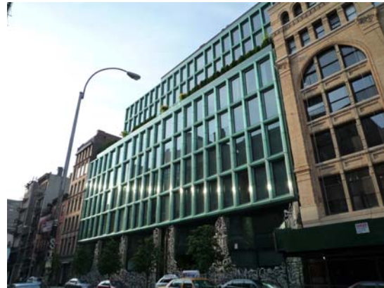
Figure 1 – 40 Bond and Neighboring Buildings
